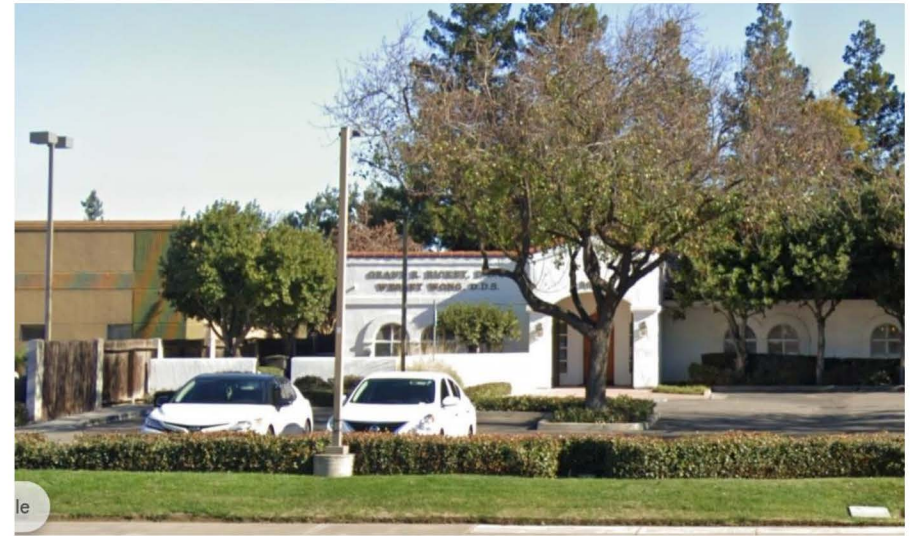
Existing Medical Clinic on site
