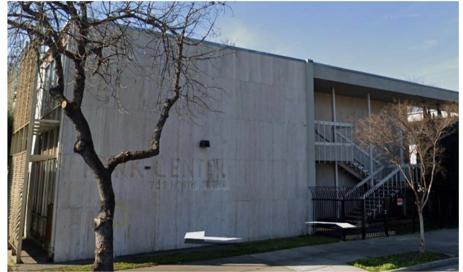
Existing Office building on-site
